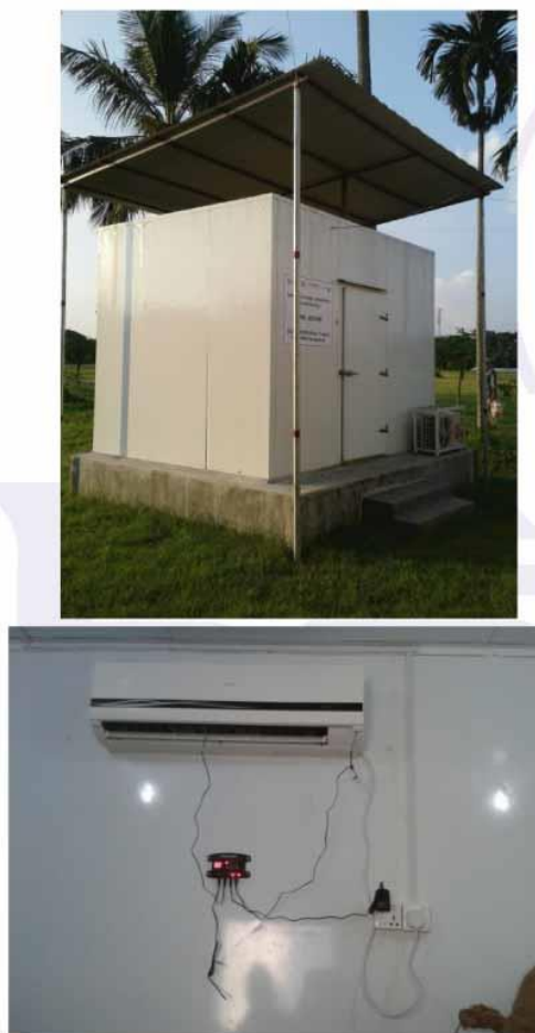
Figure 1: (Upper) CoolBot cold storage, (lower) CoolBot device connected to indoor unit of a room air cooler Image Source: USAID Horticulture Project, RARS, BARI, Jessore
